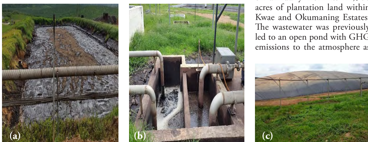
Figure 11: (a) Untreated POME wastewater from the production of 210,000 tons of oil annually is led to open ponds with emissions of GHG as a consequence. (b) The wastewater is now pumped from the refinery to the facility where biogas is harnessed. (c) The covered lagoon type biogas plant produces 18.000 m 3 biogas per day, substituting for 615 tons of diesel oil. The digestate is utilized on farmland within the plantation and local community (Ahiataku-Togobo and Owusu-Obeng, 2019).
