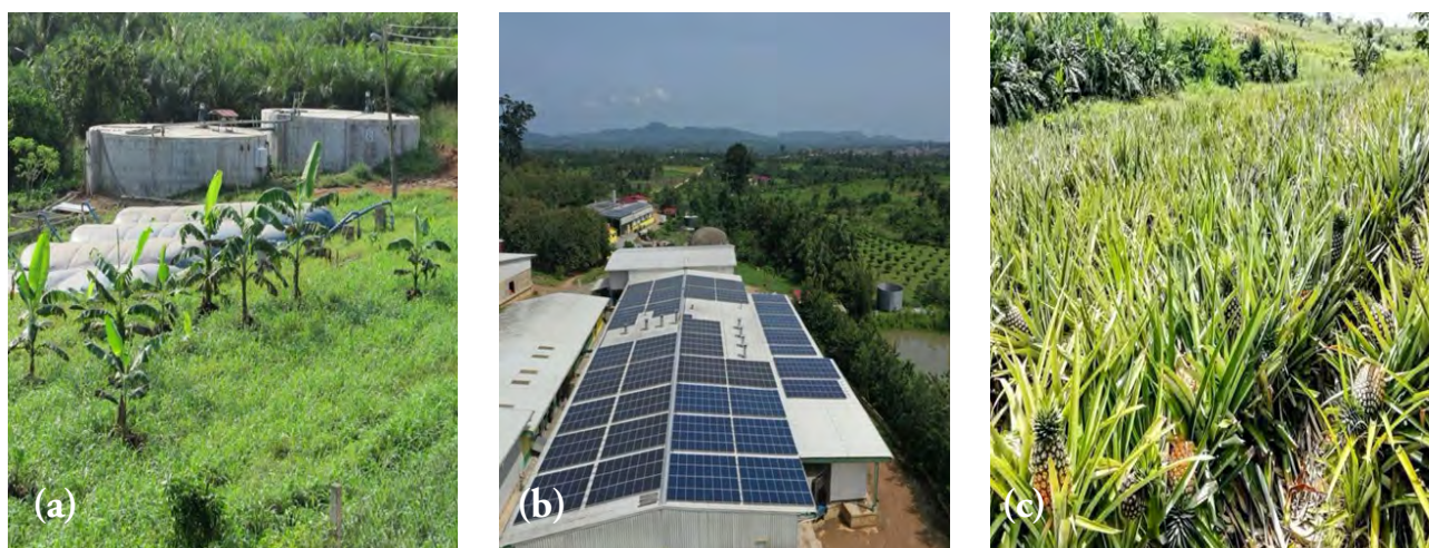
Figure 10: (a) The two 450 m 3 biodigesters constructed in concrete with balloon gas storage facilities. (b) PV installation to substitute the purchase of grid power. (c) Utilization of digestate from the company to fertilize the fruit plantations; here pineapple, as well as local farmers cropland (HPW fresh and Dry Ltd. Company, 2020)
